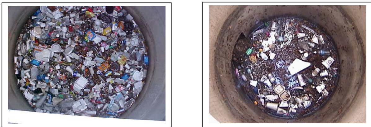
Figure 11. Gross Pollutants Captured in the CDS Units Sump
