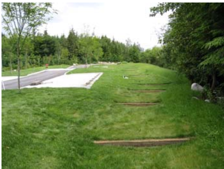
An infiltration swale located near the parking area of Crown Park in Coquitlam BC.
