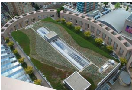
Green Roof on the Vancouver Public Library, Vancouver, BC
