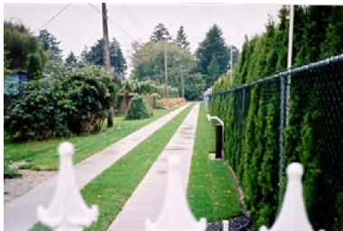
Reduced pavement in a residential lane (Source: file photo)
