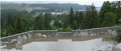
Detention Pond Overflow Weir, Sechelt
