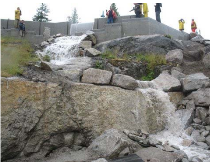
Detention Pond Overflow Weir, Sechelt
