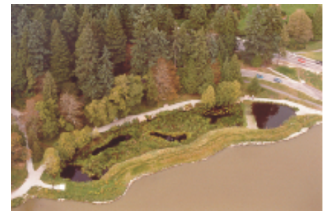
Lost Lagoon – a constructed stormwater treatment wetland located in Stanley Park, Vancouver, BC – treats road runoff from the Stanley Park Causeway which handles 60,000 vehicles per day.
