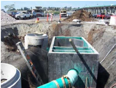
Installation of an oil and grit separator
