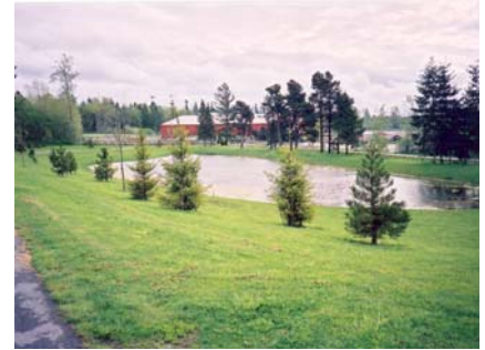
Example of a wet detention pond (Source: file photo)
