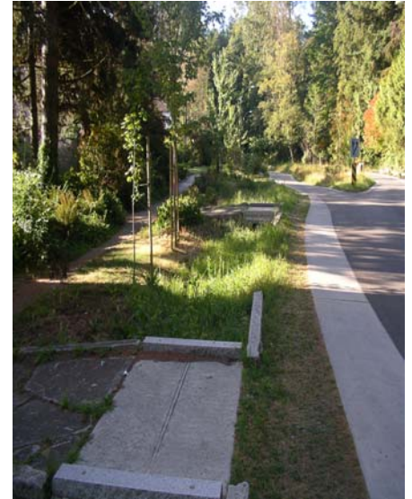
Bioswale for infiltration in Vancouver, BC
