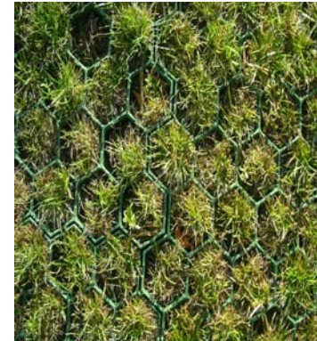
Reinforced turf, used as a pervious residential road shoulder in Vancouver, BC
