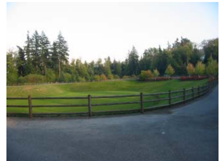
Example of a dry detention pond, WA
