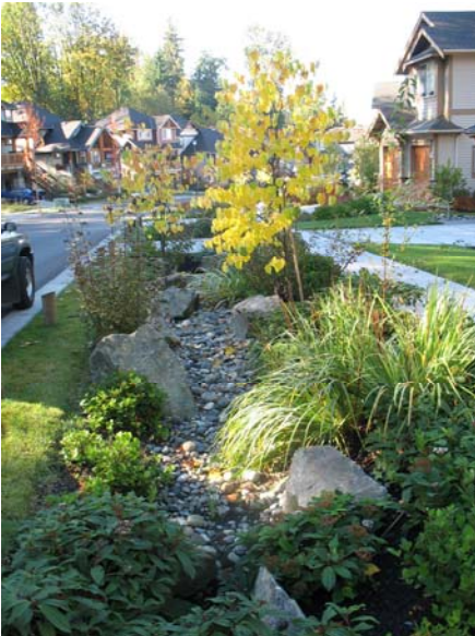
A road-side rain garden like this one in Maple Ridge, BC can help to achieve the DFO/MOE Stormwater Management Criteria for Volume Reduction and Water Quality
