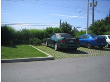
Pervious parking surface, Sechelt, BC
