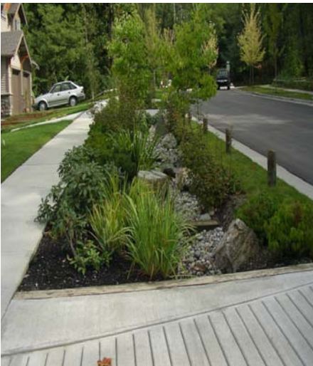
Roadside bio-retention facility, Maple Ridge, BC
