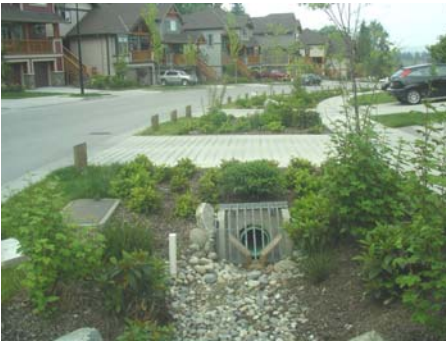
Overflow flow monitoring weir
