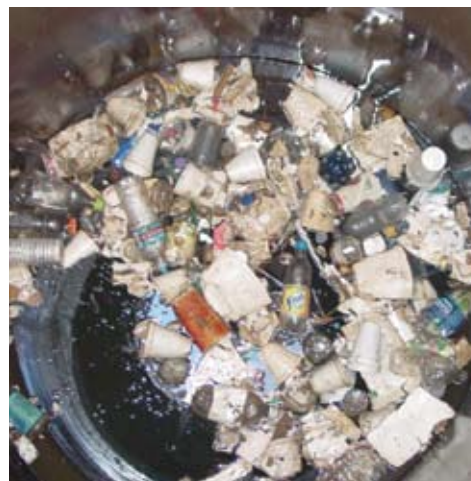
INSIDE A CDS SEPERATION CYLINDER
