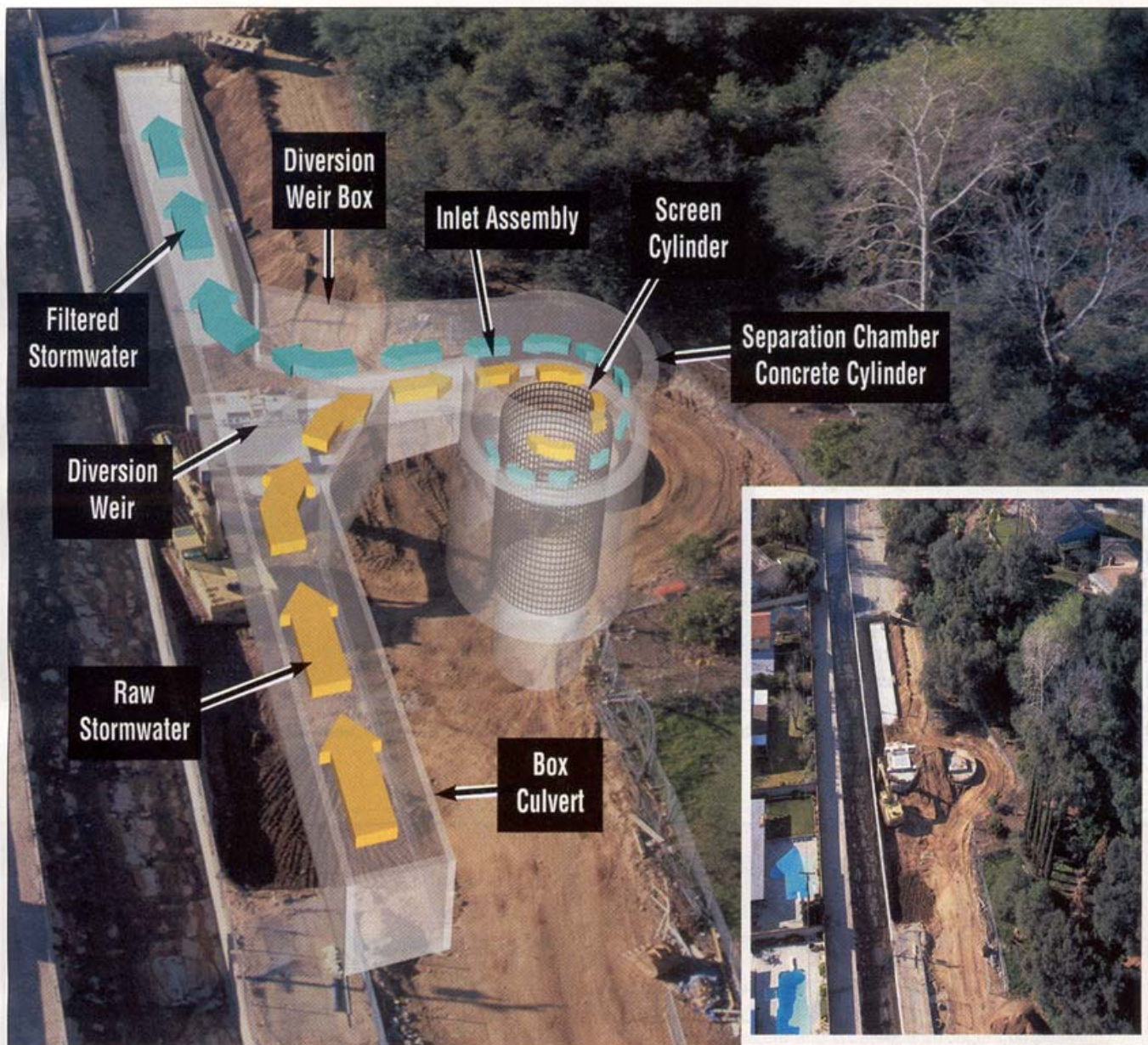
Raw storm water enters the CDS diversion chamber where a weir guides the flow into the unit's separation chamber. A vortex is formed that spins floatables and suspended solids around the screen cylinder. The screen deflects the pollutants to the center of the separation chamber. The trash and suspended solids gently settle into a sump where they remain until they are removed. The water passes through the screen, out of the separation chamber and into the diversion chamber, then re-enters the storm water flow headed downstream. Caltrans expects to have to clean the sump of this particular unit only twice a year.
